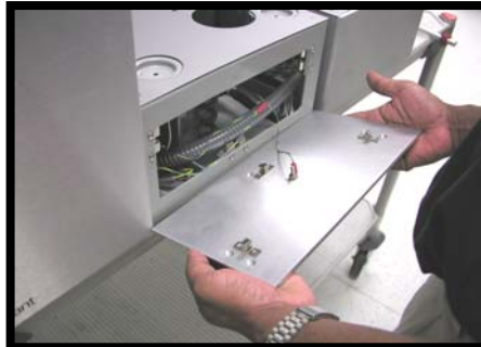
Photo 4 (Removing front panel from Cold Trap)
